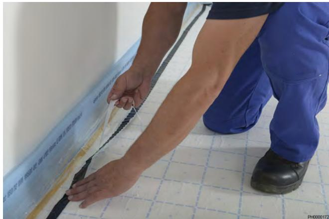
As a first step, an Uponor Multi edging strip is positioned with its rear adhesive strip to all ascending components. The laminated self-adhesive PE foil ensures the required sealing of the screed.
